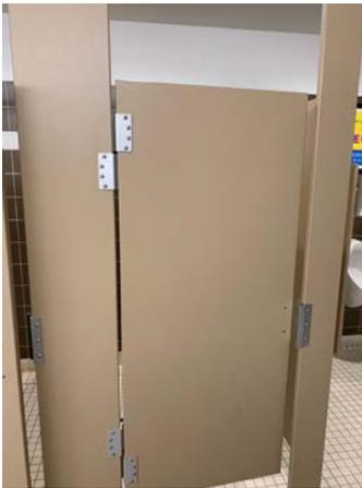
**Photo 6.2-2 Stall Doors with Gap in Front of Mirror in Trade and Tech**
