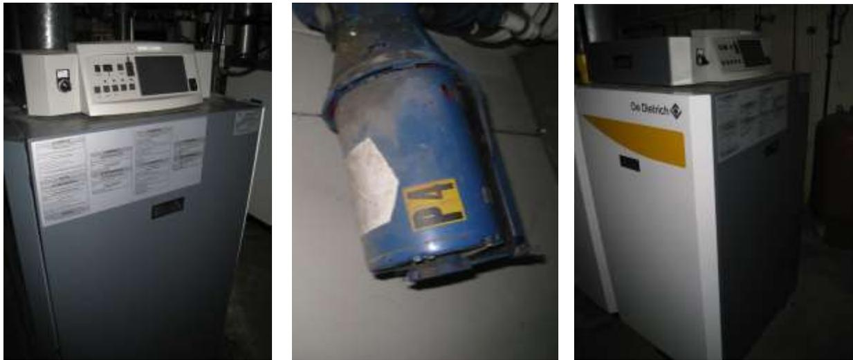
**Figure 2.7: Existing De Dietrich Natural Gas Condensing Boilers & Circulation Pump P4**
