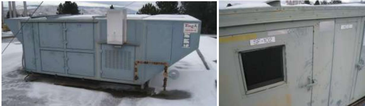
Figure 2.4: Makeup Air Unit & Air Handling Unit (SF-102)
