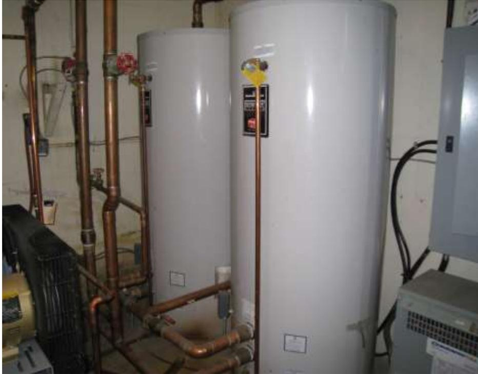
It is recommended that all HW pipework undergo an insulation retrofit.
