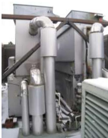
Figure 2.10: Fluid Cooler(s) located on roof
