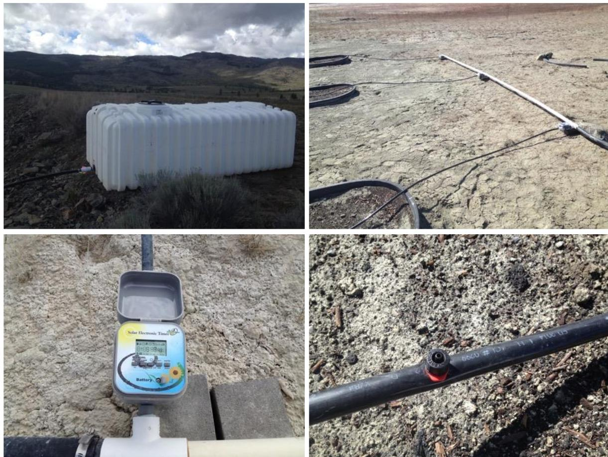
**Figure 3.6.** View of automatic gravity feed drip irrigation system installed at the Historic Afton Tailings Storage Facility research site in 2015. A 2000-gallon water tank elevated on the tailings dam (top left), 3-way independent water delivery system (top right), low pressure automatic irrigation timer (bottom left) and  $\frac{1}{2}$  gallon/hr. drip nozzle (bottom right).
