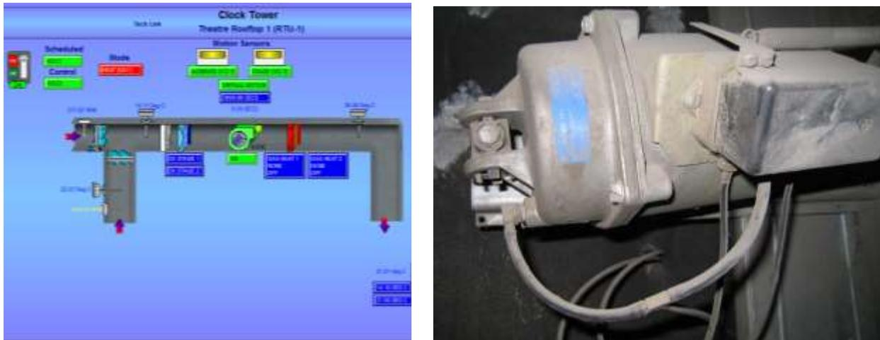
**Figure 2.6: Theatre Rooftop Unit – DDC Graphic & compressed air damper actuator**
