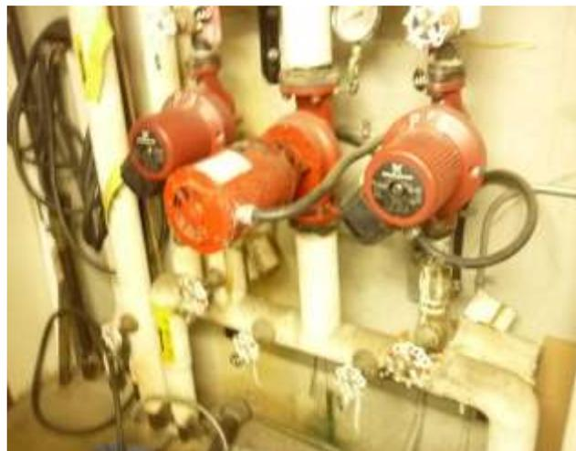
Figure 2.5: Hot water boilers and hot water distribution pumps
