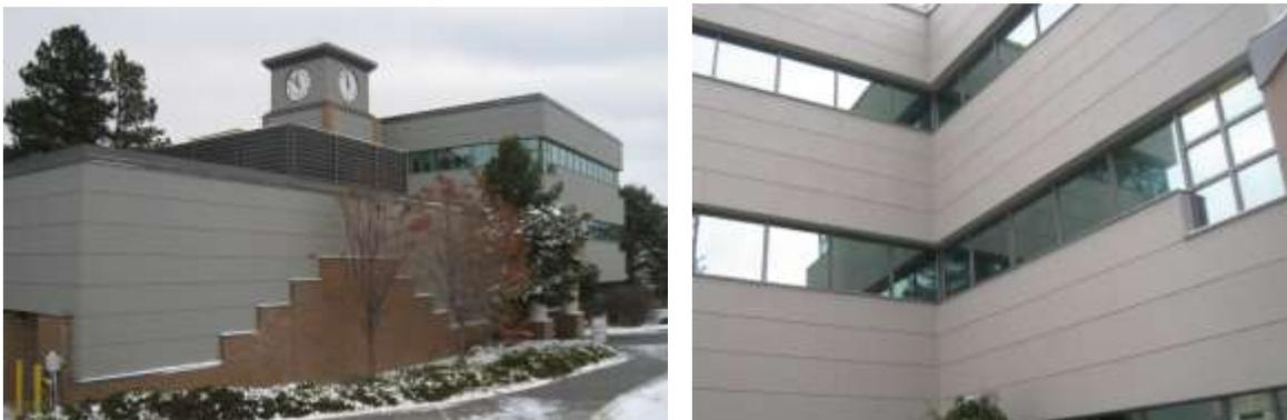
Figure 2.1: Building Envelope & Glazing Units
