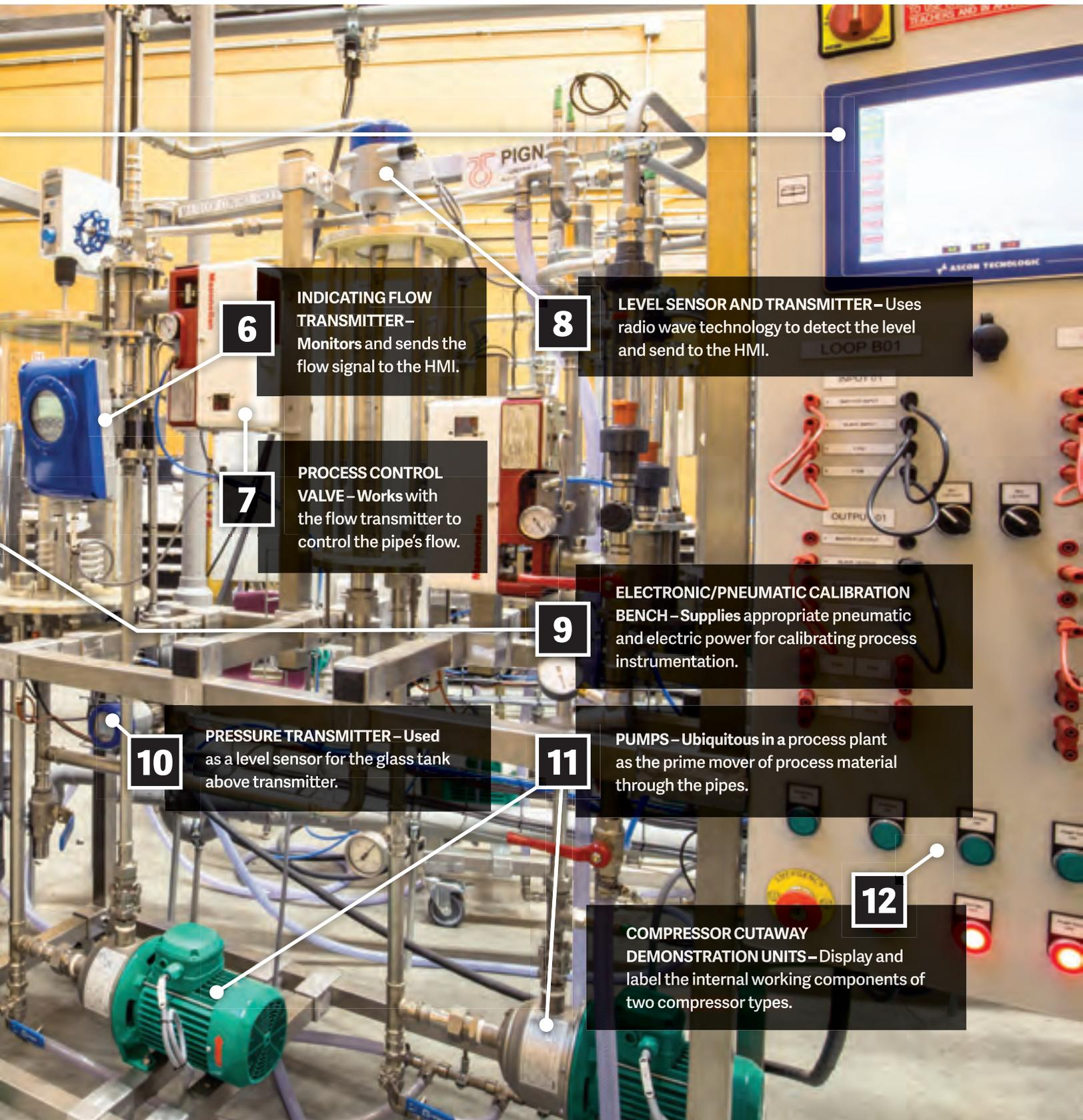
**6** **INDICATING FLOW TRANSMITTER** – Monitors and sends the flow signal to the HMI.
