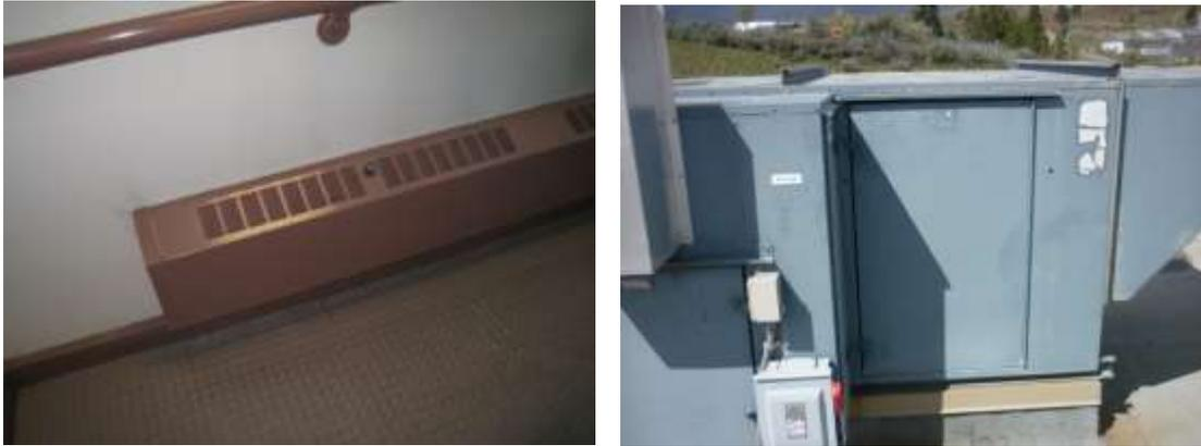
Figure 2.6 Baseboard Heater and Gas Fired RTU
